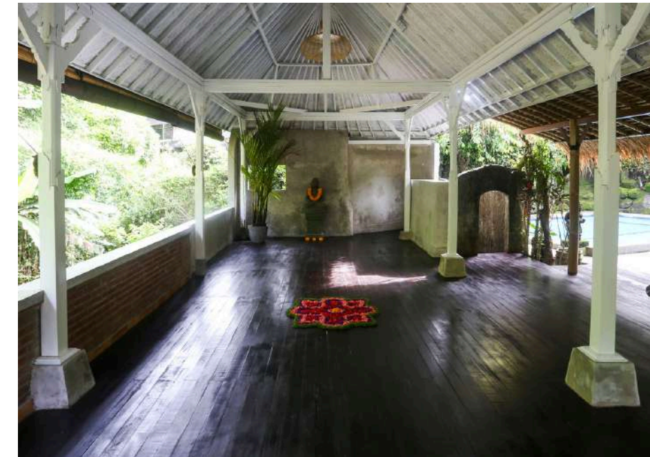
Water Shala – Built over a river in the heart of Ubud, surrounded by green plants for a peaceful and relaxing atmosphere.
